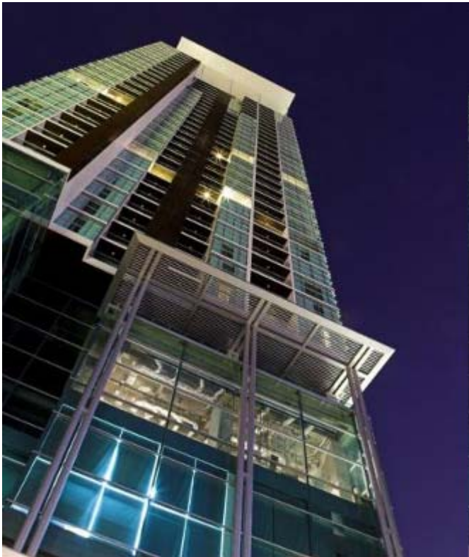
Fraser Suites Serviced Apartments
